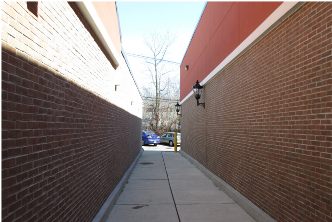
Existing Walkway between Buildings
