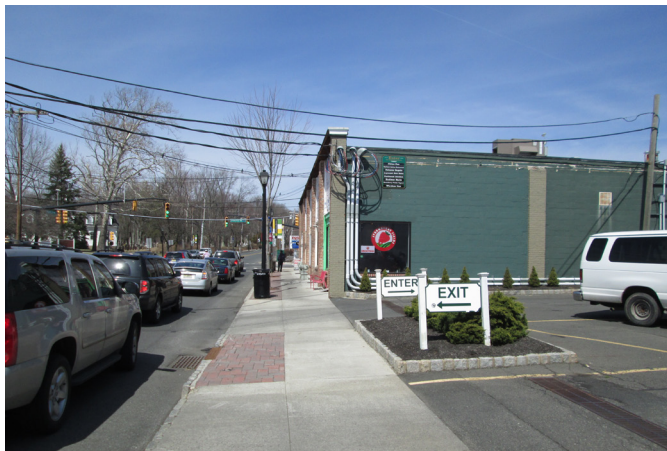
Curb Cuts Along South Street
