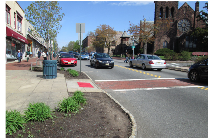
Curb Bump-out in S. Orange
